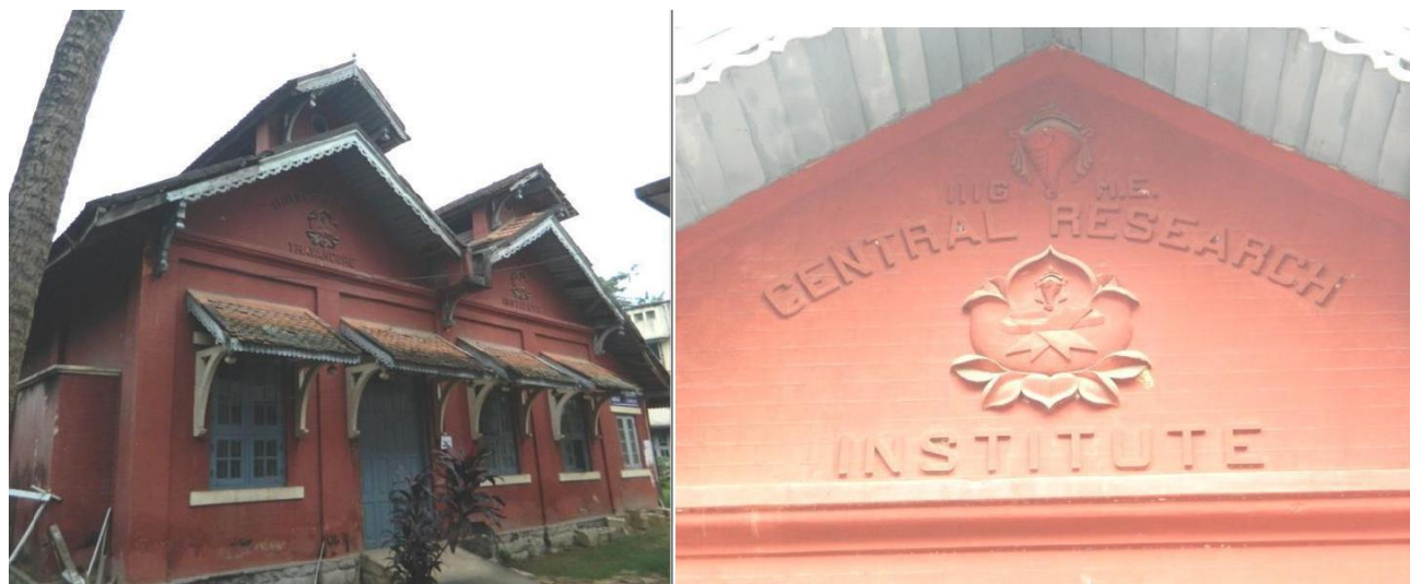
Fig. 3.1. Buildings in the Central Research Institute of University of Travancore
