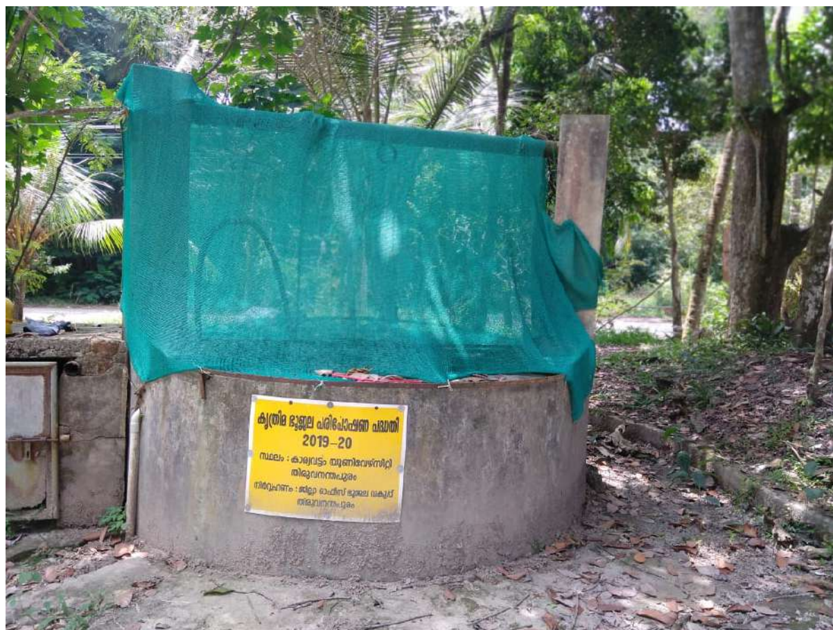
Figure 3. Roof top recharge well (courtesy: Prof Rajesh Reghunath).
