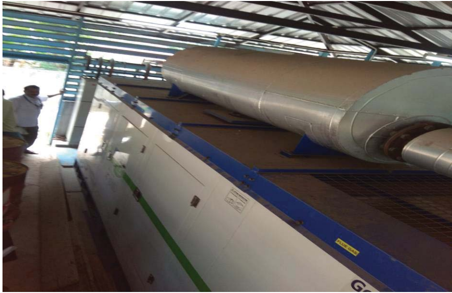
Top side of the DG Set
