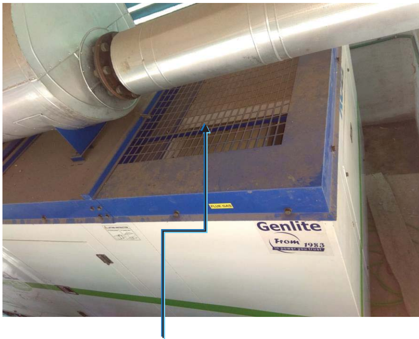
Hot air passes through this portion
